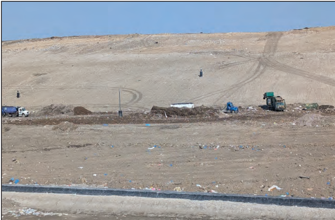
Phase 4 viewed from the East
