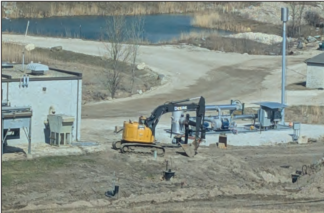
Construction of new flare, adjacent to Gas Plant
