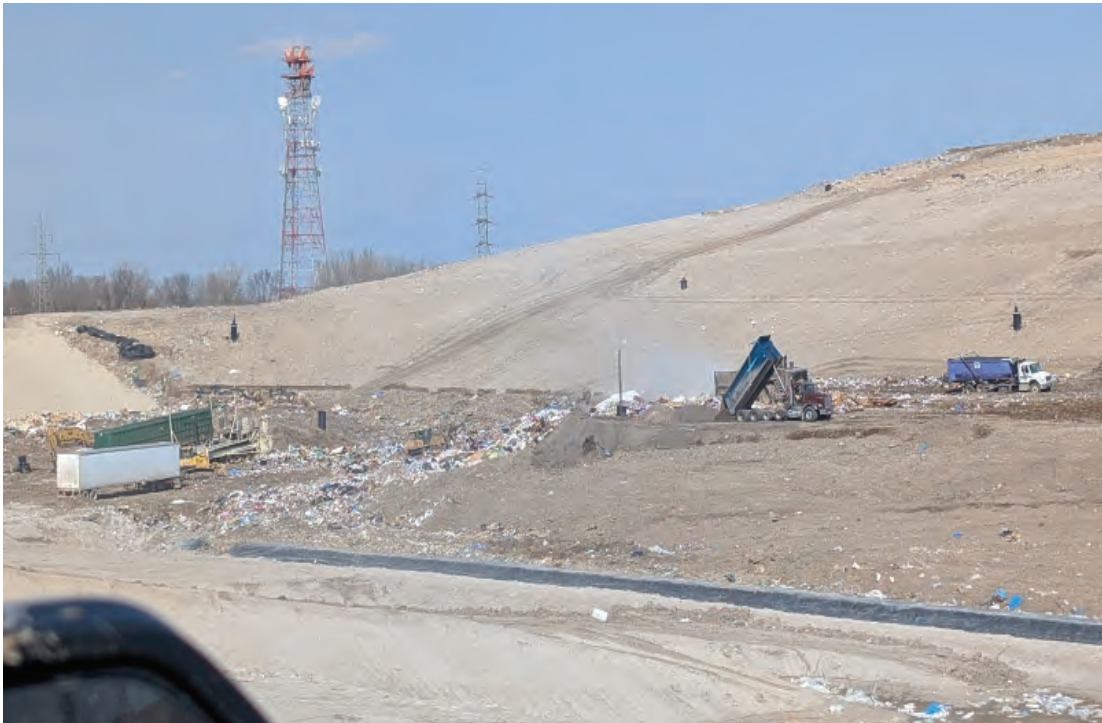
Tipping into previous access road into Phase 4
