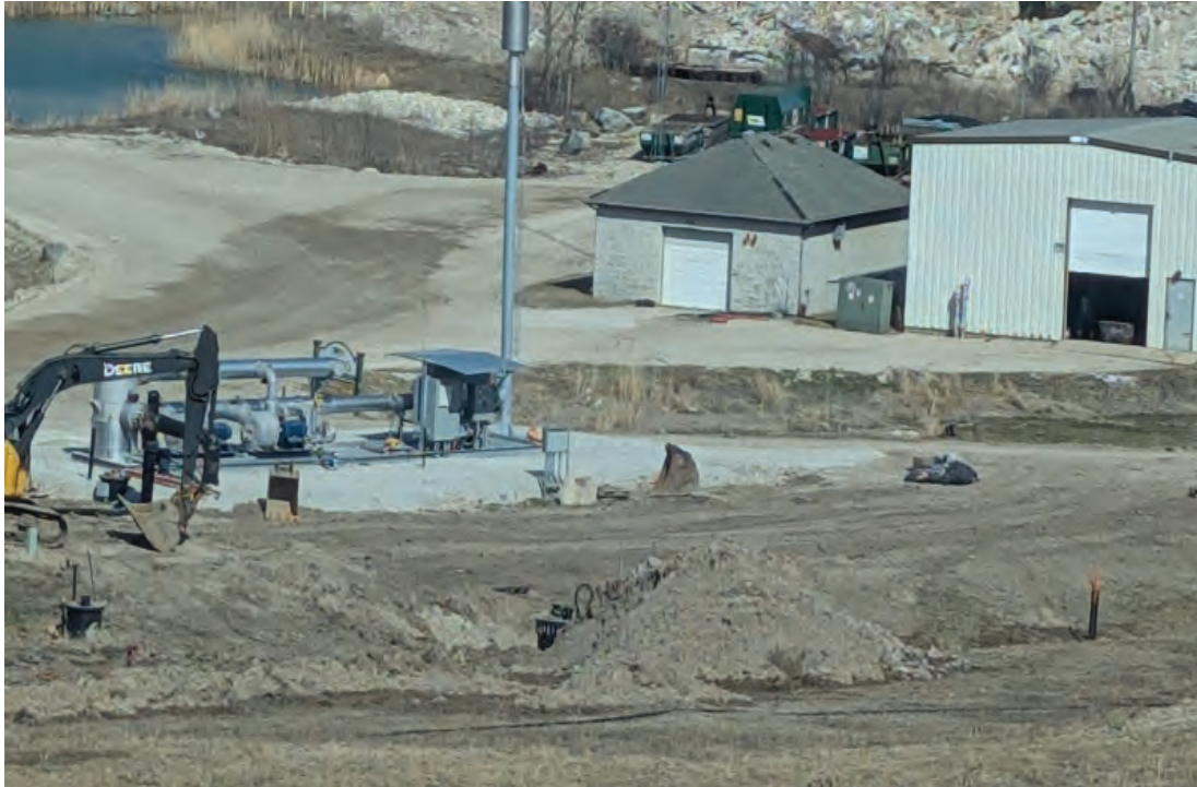
North end of PhasConstruction of new flare
