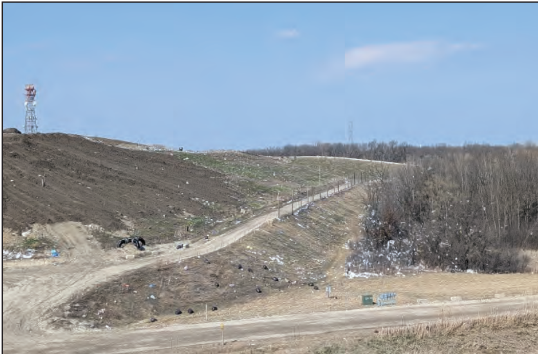
East slope of Phase 1, top soil cover nearly complete
