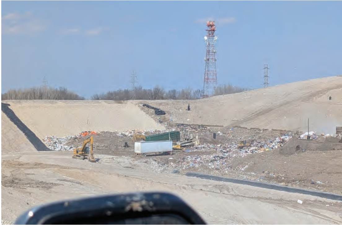
Tipper set sideways/East-Weat in Phase 4
