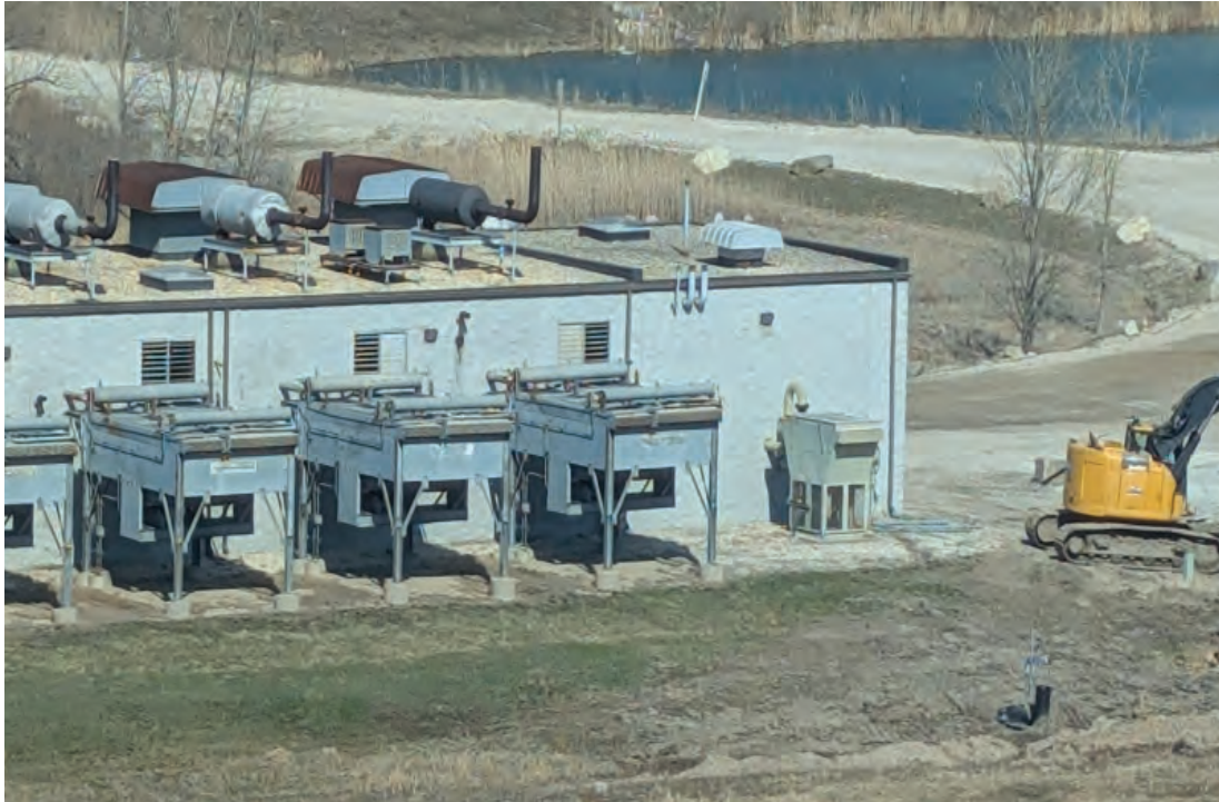
Energy/Gas plant, adjacent to new flare construction
