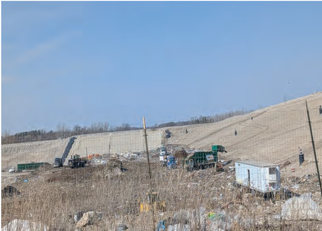
Trucks cleaning out against Phase 3, from Phase 4
